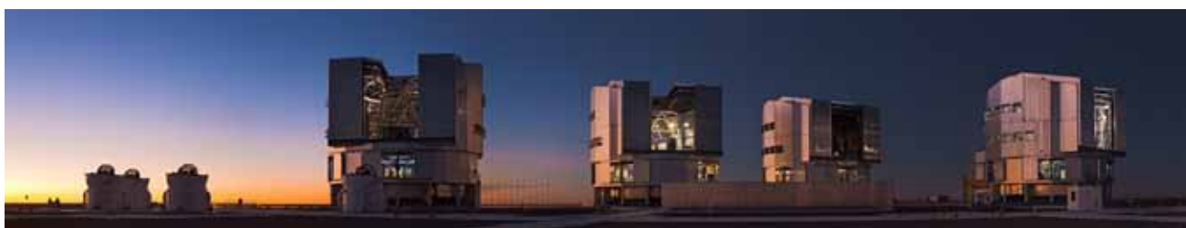
The Very Large Telescope system shortly after sunset. During daytime, the huge telescope structures are cooled to the air temperature forecast by ECMWF. The people who can be seen on the left provide a sense of scale. Photo: ESO/B. Tafreshi (twanight.org)
